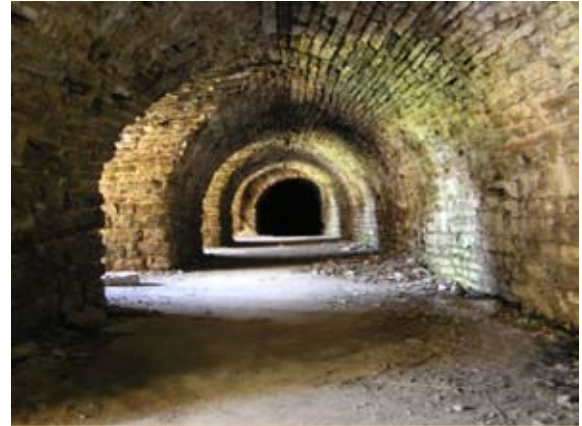
A vaulted casemate in the Honor Bastion.
